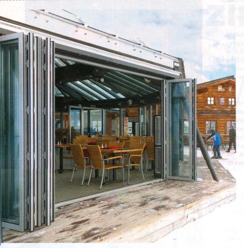
NanaWall. The SL70 thermally broken aluminum-framed folding glass wall system is now
