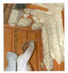
CertaSpray foam insulation from CertainTeed Corp. is offered in open- and closed-cell formulas. The product creates an air seal and can be used alone or with fiberglass insulation. The open-cell formula expands to create a soft, flexible insulation, and the closed-cell formula results in a hard, rigid consistency that provides added structural integrity.
