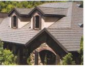
Vail Titan Select metal shingles by Custom-Bilt Metals are made with heavy-gauge metal construction and an interlocking design making it nearly impossible for moisture to penetrate. The shingles reflect up to 70 percent of the sun's energy. For more info circle #42
