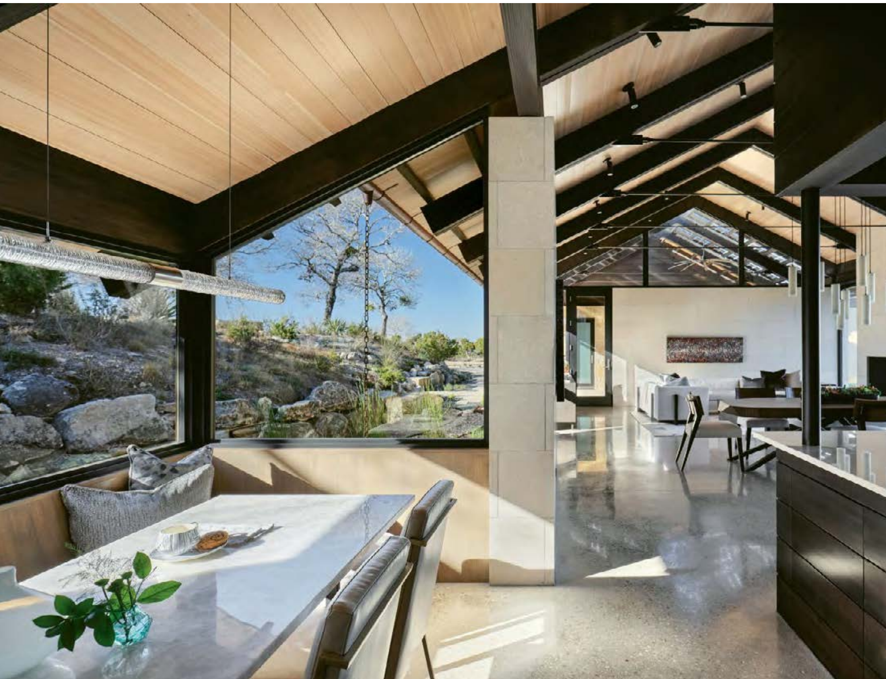
This page: In the great room, dark-stained framing contrasts with honed limestone walls and terrazzo-like concrete floors. The specks of color in the floor come from the Medina river rock aggregate used in the pour. Ceilings are hemlock with a transparent white glaze to preserve the evenness of the finish.
