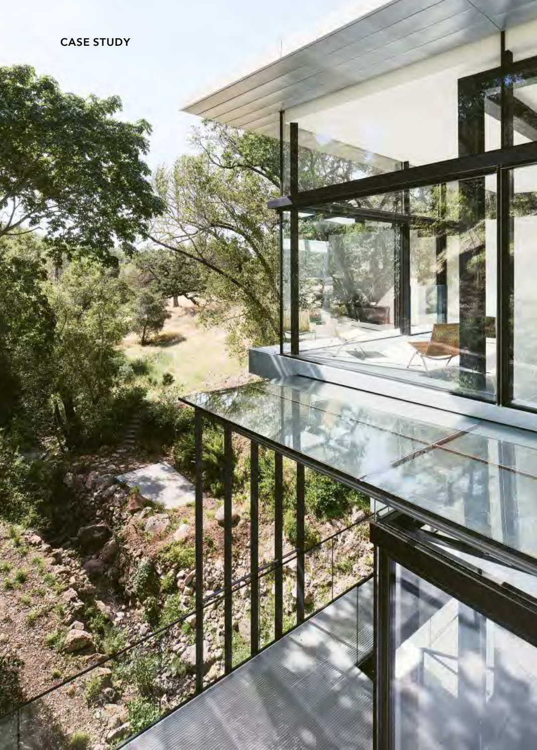
The steel superstructure is bolted into the creek banks, entirely suspended on steel caissons and 3¼-inch rods drilled horizontally into the stone.
