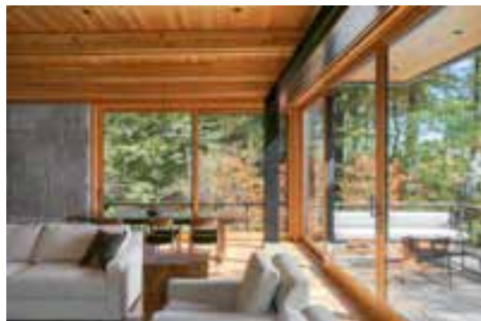
Black painted steel threads through an interior of large-format granite masonry and Douglas fir glulam beams and walls.
